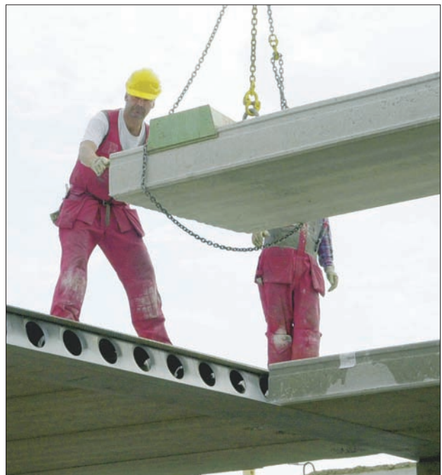
Figure 4 Floor slabs craned into position
