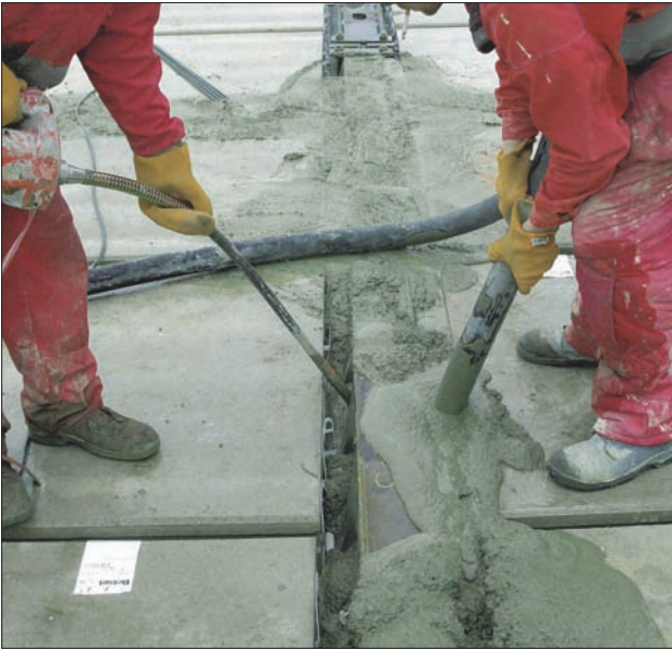
Figure 5 Placing concrete
