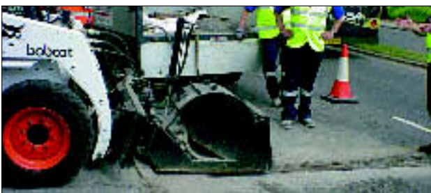
Figure 1 Mechanical planing-out of cracks
