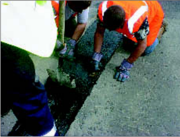
Figure 4 Application of Permatrack H
