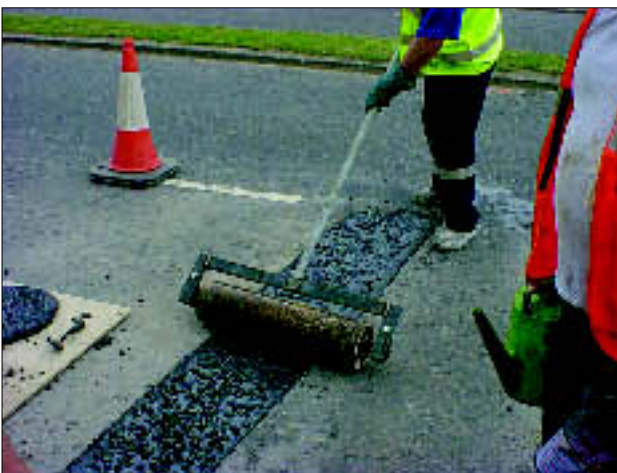
Figure 5 Rolling-in pre-coated chippings
