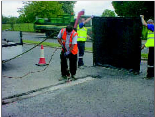
Figure 2 Drying and cleaning the recess
