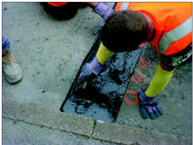
Figure 3 Application of Permatrack PSB to recess
