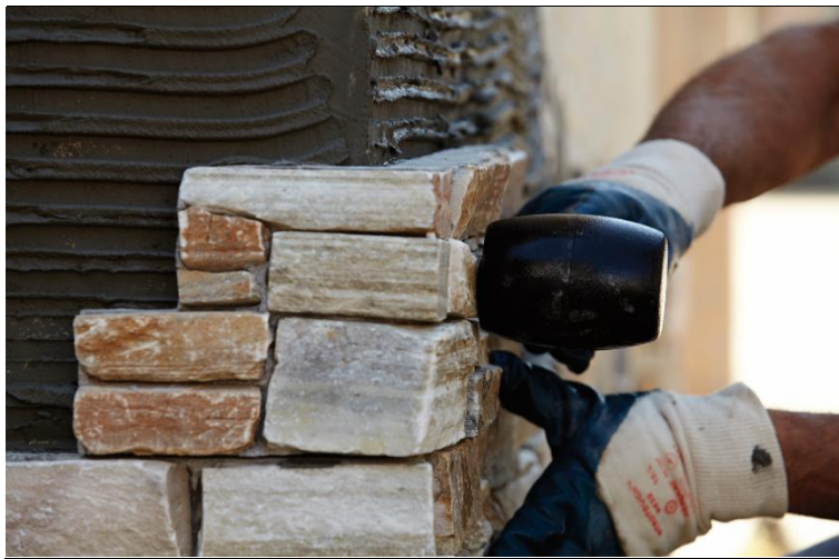
Figure 5 Stone panels bonded to the wall
