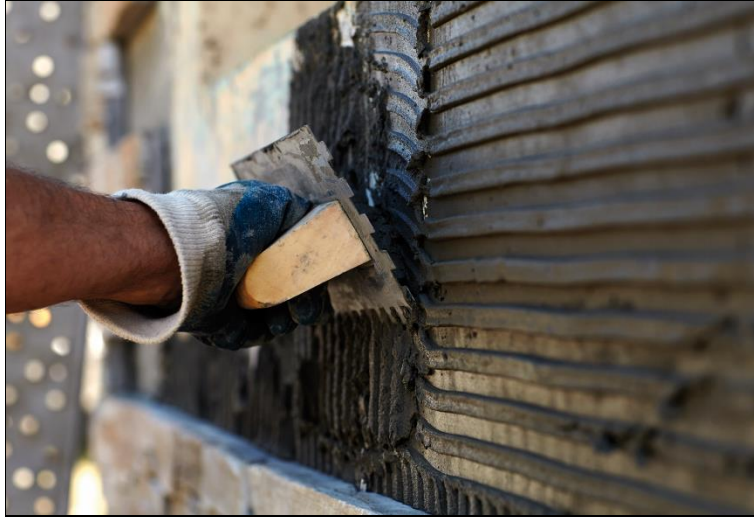
Figure 5 Stone panels bonded to the wall
