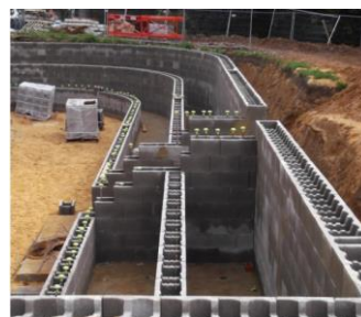
Cert: 20/5774 Anderton Concrete Products Structural shuttering block system
