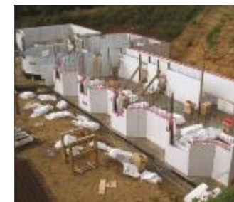
Cert: 06/4347 Quad-Lock Building Systems Insulating concrete formwork (ICF) system
