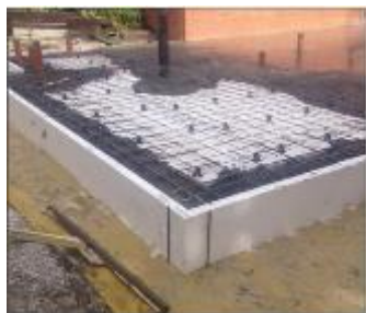
Cert: 19/5617 Build-Lite Foundation system using EPS insulation & reinforced concrete
